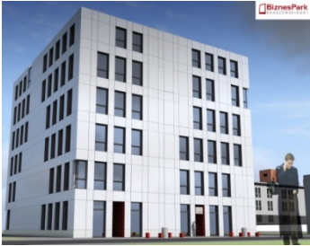
Biznes Park at 1 Kraszewskiego Street - area: 21 000 sqm
